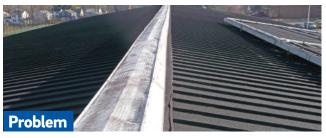
The roof on this ice rink had been covered with an asphaltic product that was delaminating from the metal roof it was intended to fix. An abandoned hot water heating system was corroding and causing leaks into the building. To compound things, the building was inadequately insulated and had ventilation problems. All of these items contributed to an unsafe and undesirable skating environment.
