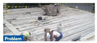
An antiquated design in pre-engineered buildings called broached endwalls reduced the slope of the roof to nearly flat at the endwalls resulting in premature corrosion of the roof panels.
