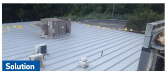
The Butler Slope Build-Up Reroof System coupled with the High-Profile Metal-Over-Metal Retrofit System allowed the contractor to increase the slope at the endwalls thus creating a consistent roof plane to ensure long-term performance from the new MR-24<sup>®</sup> roof.
