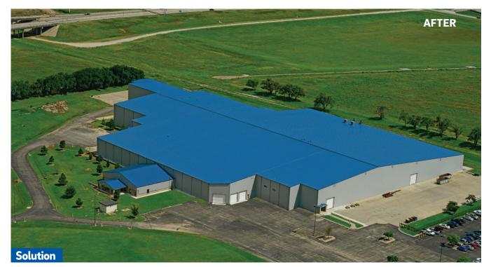
XLT Ovens conducted a review of available products and systems and chose a Butler<sup>®</sup> solution based on its proven performance characteristics. Butler's solution included the Slope-Build Up Retrofit system utilizing the MR-24<sup>®</sup> roof system which allowed for expedient installation right over the existing roof with minimal interruptions to their business.
