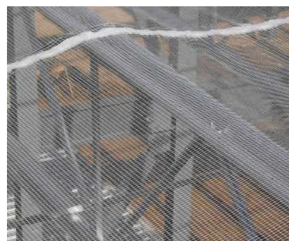
Sky-Web® and Sky-Web II® do not eliminate fall hazard from the non-leading-edge perimeter of the roof during installation.
